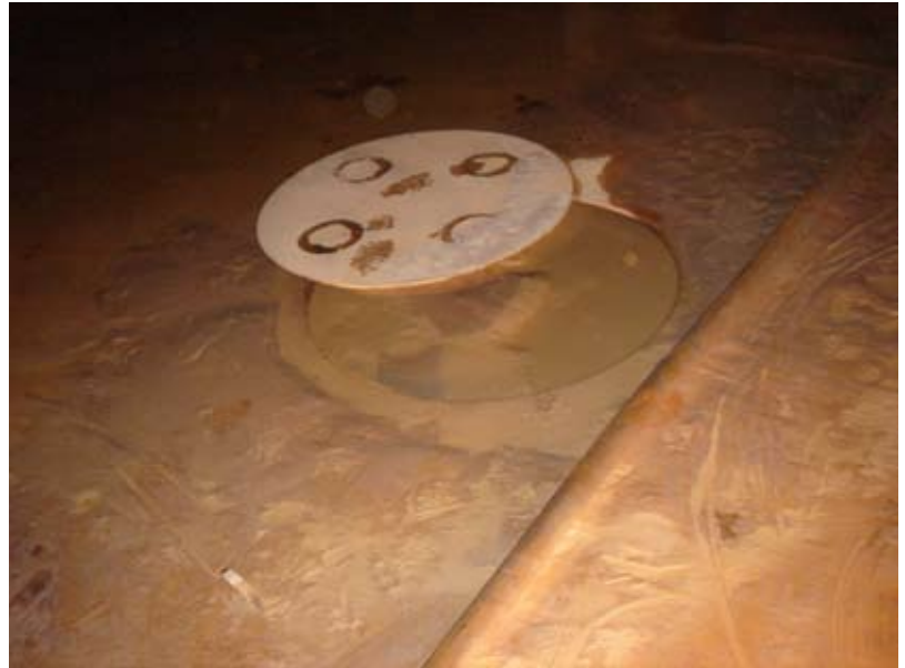
AK Services safely cut holes in the floor of a leaking petroleum tank so contaminated sand could be removed from beneath the tank. Photo courtesy AK Services
