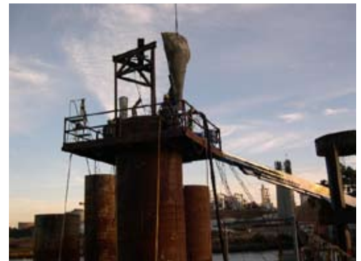
Bridge contractor Kiewit hired AK Services to remove 13 pilings that were mangled by stubborn bedrock. AK cut 3,500 linear feet of steel, working in a caisson 150’ below sea level. Photos Courtesy AK Services
