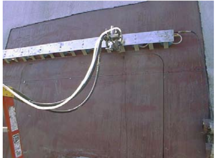
Cutting a door sheet in a petroleum tank. Waterjet is commonly used for this application because it cuts without flames or heat. Photo courtesy AK Services
