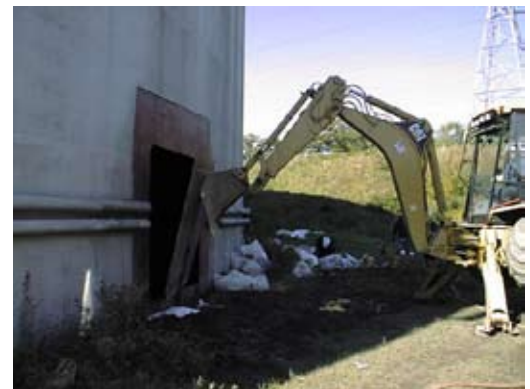
Cutting a door sheet in a petroleum tank. Waterjet is commonly used for this application because it cuts without flames or heat. Photo courtesy AK Services
